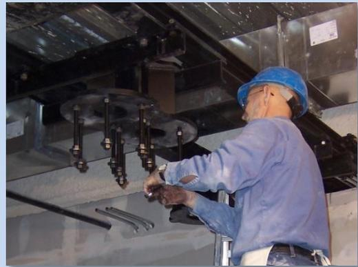
At UK Chandler Hospital's new patient pavilion, HTC provided a total of 153 Accu-Mount Support Systems, designed to attach to both the steel and concrete form building structures. The support systems were supplied for a vast majority of equipment weights, moments and types and included mounts for tandem ICU booms, single equipment booms, anesthesia booms, surgical lights, exam lights and flat panel monitors.
